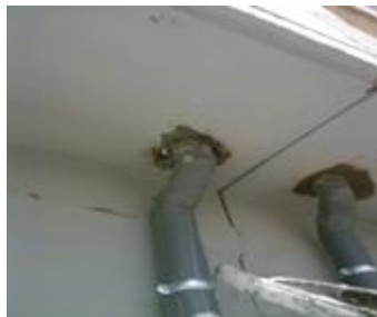
photo 10: Placing “PVC” Tube for evacuating Balcony Waters
