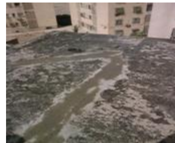
photo 11: Replacing the Old Covering by “pax” with
