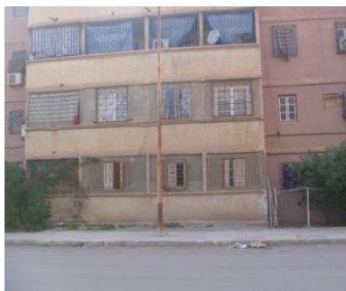
Photo 2: Adding frames of steel for windows and balconies Source: Author in 2015
