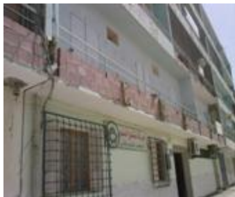
Photo 09: Building Balconies with Bricks
