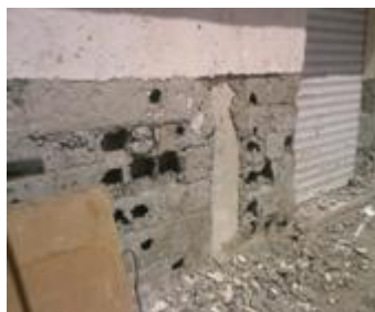
Photo 12: removing the old outdoor covering with well cleaning and covering the walls with Cement type “Térolliane”
