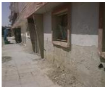
Photo 12: removing the old outdoor covering with well cleaning and covering the walls with Cement type “Térolliane”
